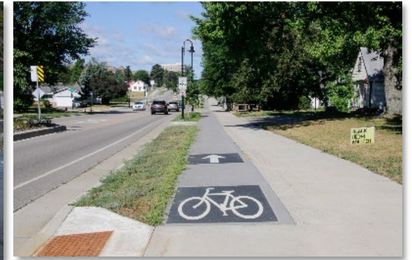
▲ Curb separated directional (one way) cycle track adjacent to sidewalk. (Richfield, MN)
