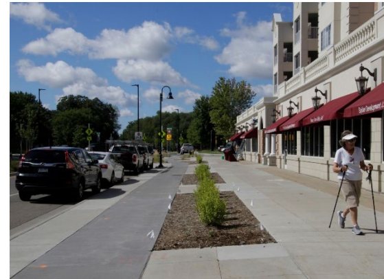
▲ Curb separated cycle track with landscaped buffer space between the protected bike lane and sidewalk. (Richfield, MN)
