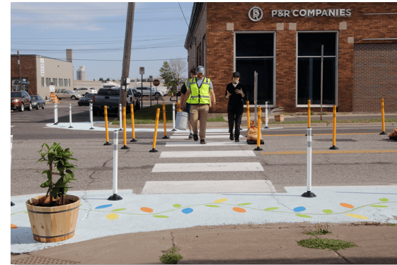
▲ Temporary curb extensions create space for community to paint the pavement, adding visual interest. (Duluth, MN)
